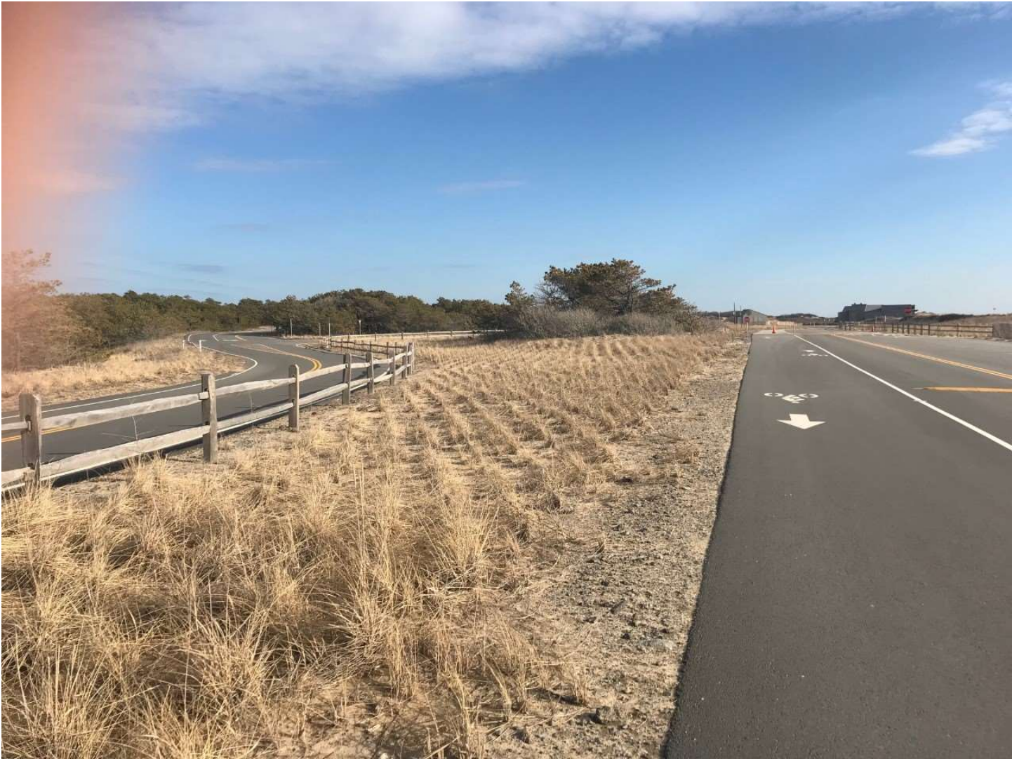
End of Route 6 trail - proposed connection to existing parking lot/bike path
