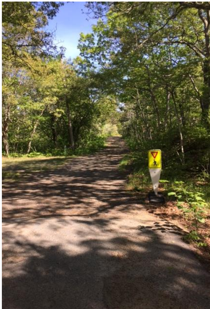
Flexible in-street pedestrian crossing along Old Colony Trail
