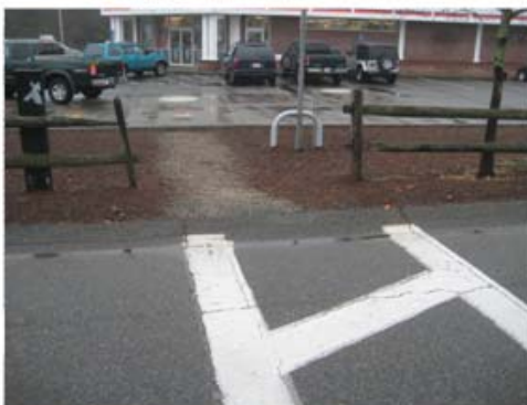
Crosswalk on the north end of Shank Painter Road, looking westbound at the Cumberland Farms parking lot. The path from the sidewalk beside TD Bank across to Cumberland Farms is not handicap accessible, requiring patrons to traverse an off-road path then overcome a curb onto the lot.
